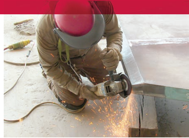
Grinding on a platform for weld preparation.
